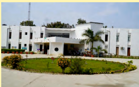
Admin Office & Research Centre
