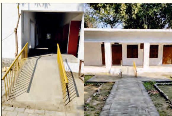
Ramps for Easy Access to Classrooms
